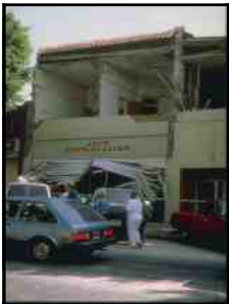
[Uptown Earthquake Damage]
